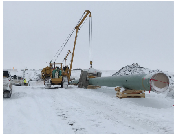
16. Off side welding – km 109+50 – Nov 17, 2017
