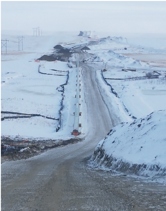
11. Waiting to lower pipe – km 68+400 – Nov 15, 2017
