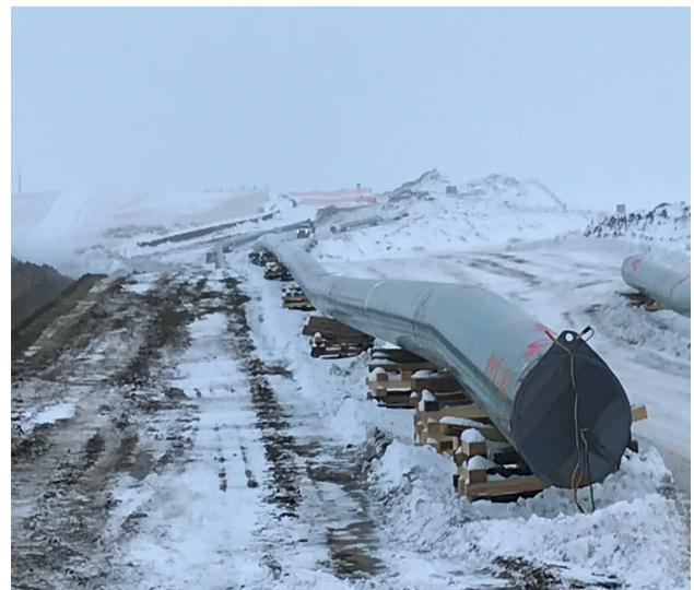
4. Welded pipe on skids – Km 68+400 – Nov 13, 2017
