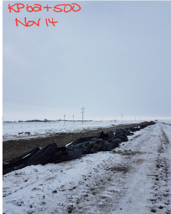
10. Pipe in the ground – km 62+500- Nov 14, 2017
