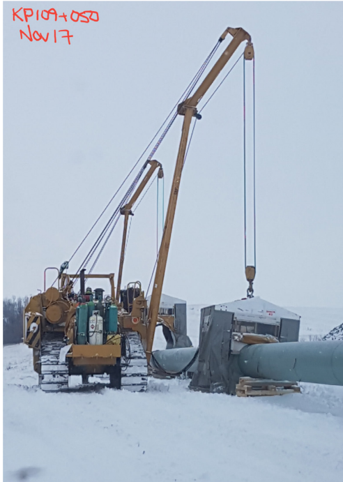
17. Off side welding – Km109+50 – Nov 17, 2017
