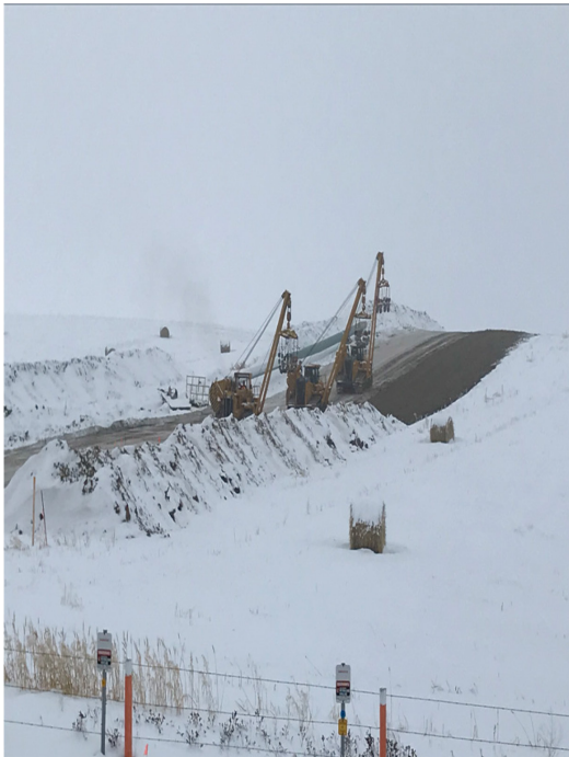
3. Lowering-in Crew – Km64+550 – Nov 13, 2017
