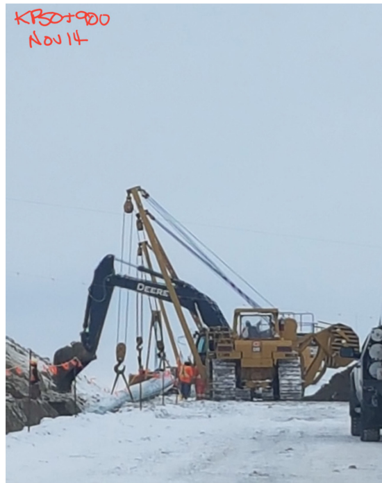
8. Pipe lowering – Km 50+900 – Nov 14, 2017
