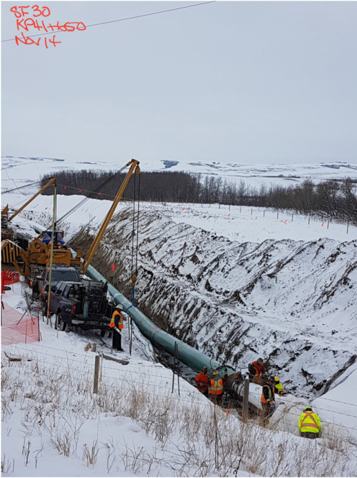
5. Tie-in – Km 41+650 – Nov 14, 2017
