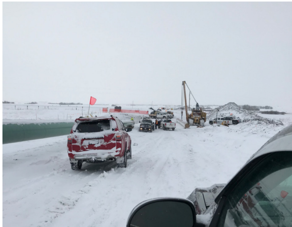
15. Tie-in – Km 81+450 – Nov 17, 2017
