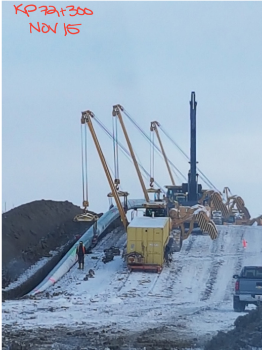
13. Pipe lowering – km 72+300 – Nov 15, 2017
