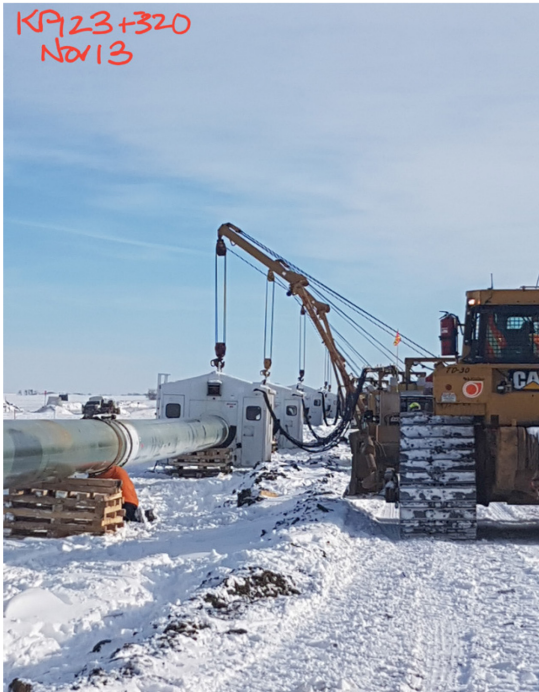
1. Welding Crew – Km123+320 – Nov 13, 2017
