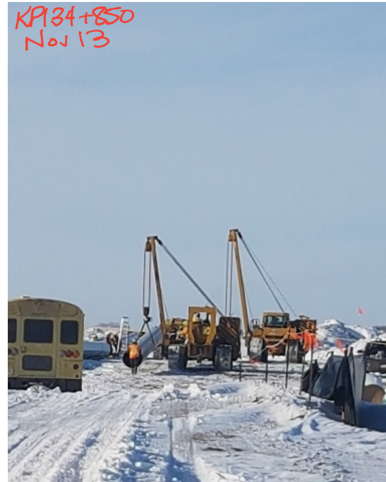
2. Bending Crew – Km 134+850 – Nov 13, 2017
